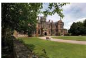
Ingestre Hall (IH) - an expressive arts centre set in a wonderful Staffordshire Jacobean mansion.
